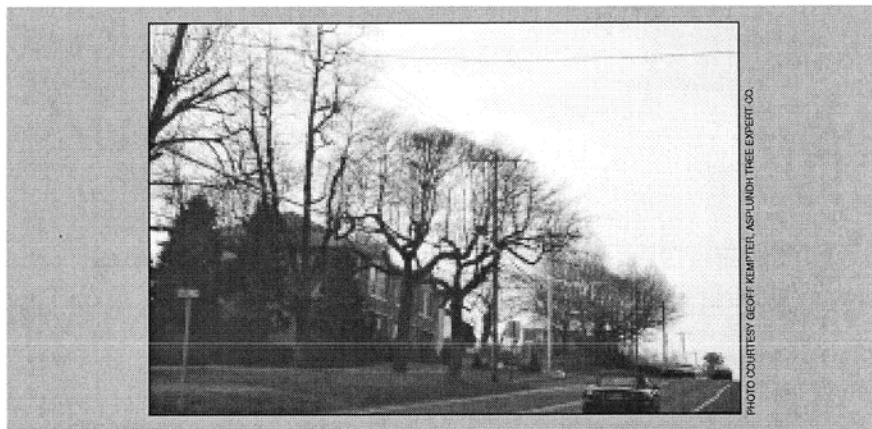
Fig. 5. Trees under these wires were topped improperly several years ago. Vigorous regrowth of slender branches from the stubs of thicker branches grew into the wires, requiring pruning for clearance.
