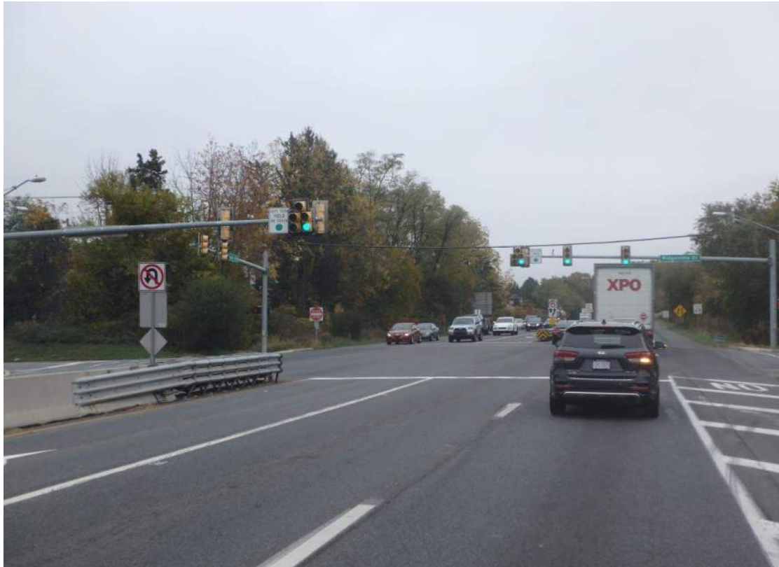
Direction / Road: NB Route 309 Approach / Departure: Approach Distance: 50 feet
