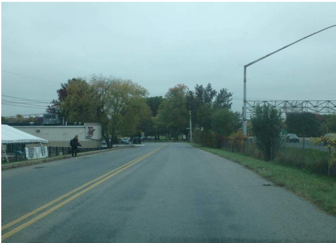
Direction / Road: SB Bulldog Drive Approach / Departure: Approach Distance: 150 Feet
