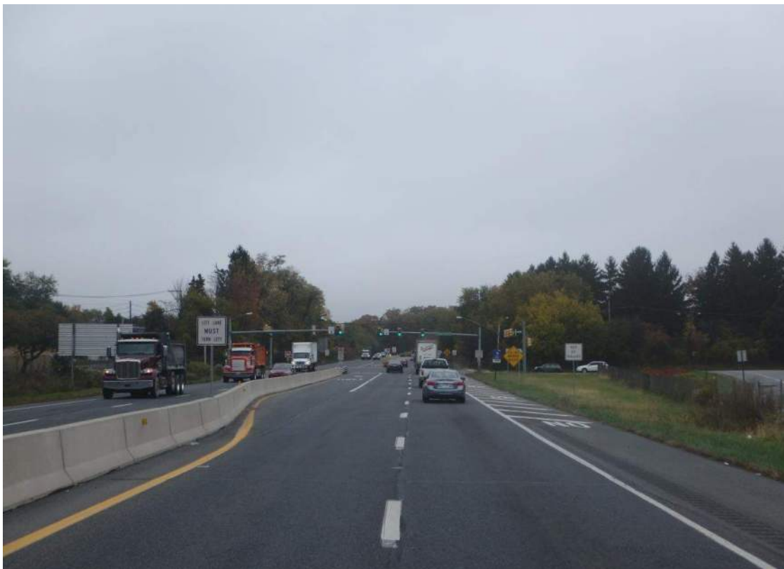
Direction / Road: NB Route 309 Approach / Departure: Approach Distance: 150 Feet
