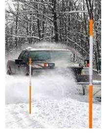
If installed correctly this will help with winter operations. If followed correctly snowplows will not hit them with the corner of the plow and the roll of snow coming off the plow will not knock it down.
