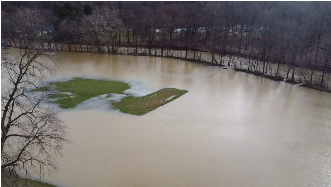
Jordan Creek Flooding | Source: South Whitehall Township
