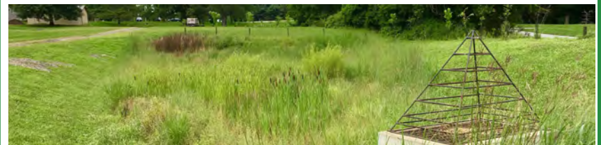
Bioretention Basin | Source: Hillendale Elementary School
