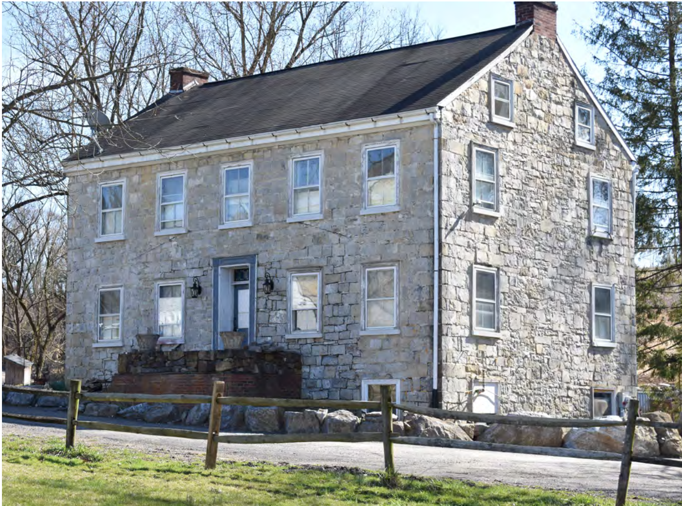
1800 Adam Good (Guth) Home | Source: South Whitehall Township
