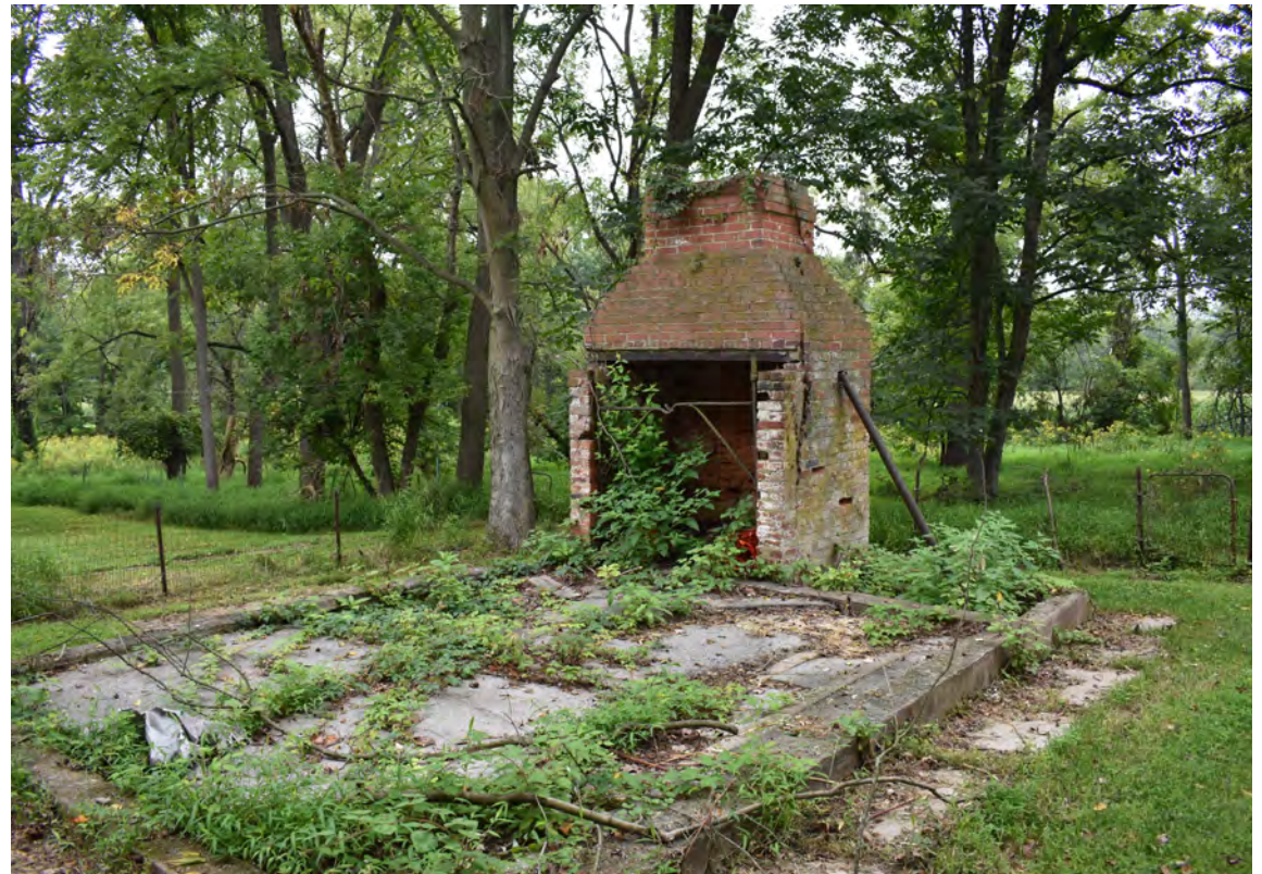
Remnants of an old outdoor oven / Source: South Whitehall Township
