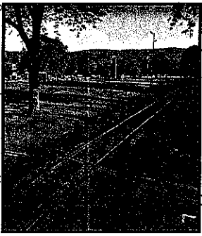
EXAMPLE OF CONCRETE SIDEWALK TRANSITIONING TO ASPHALT PAVING TO CROSS RAILWAY
