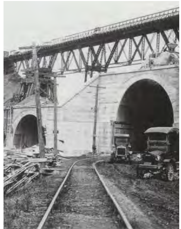
Construction of the Iron Bridge
