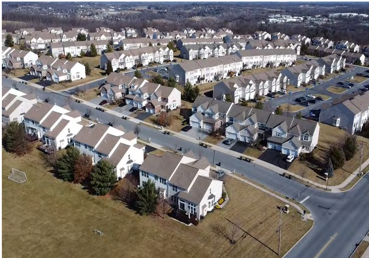
The Vistas at Green Hills
