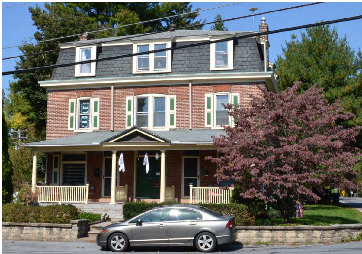
Multi-Unit Apartment in Greenawalds
