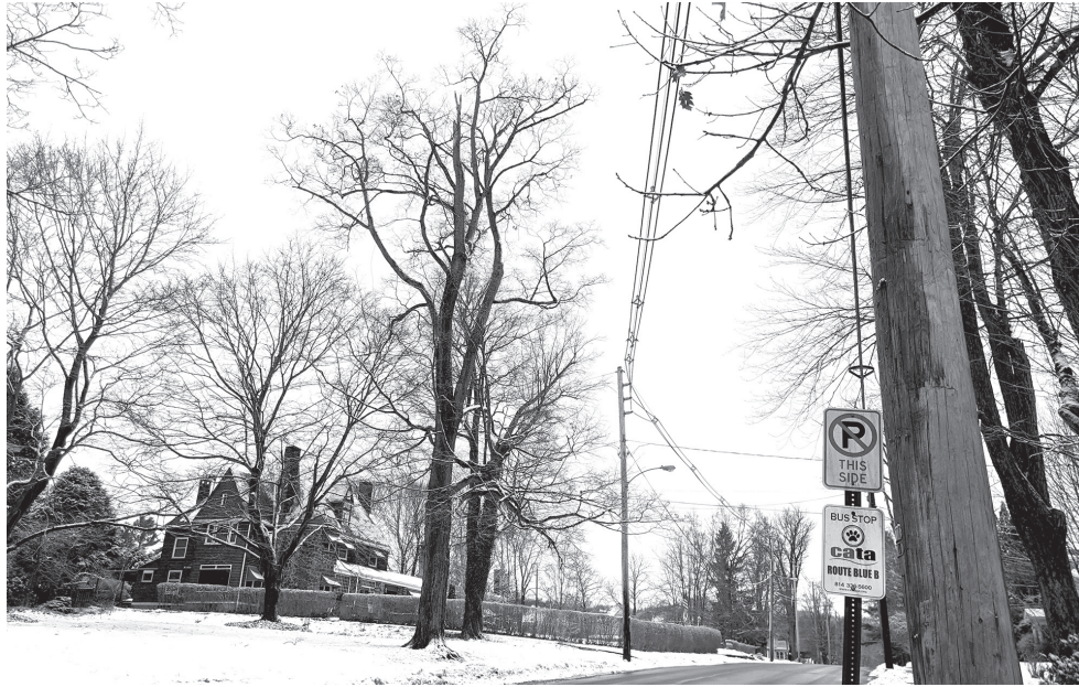
Figure 6. To safely clear the conductors mounted on the utility cross-arm, all tree scaffold limbs were pruned from the side toward the street. All branches likely to grow back over the lines were pruned to avoid regrowth from falling onto the lines during winter ice storms.
