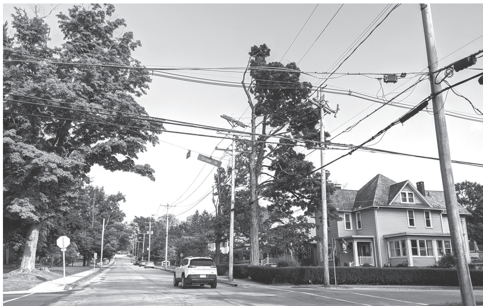
Figure 7. The trees at the left side of this photo were pruned to clear high-voltage conductors. A large limb growing at the right side of the nearest tree was pruned to lateral, which remains growing away from the line. This retains the tree's natural shape and provides long-term safe clearance.
