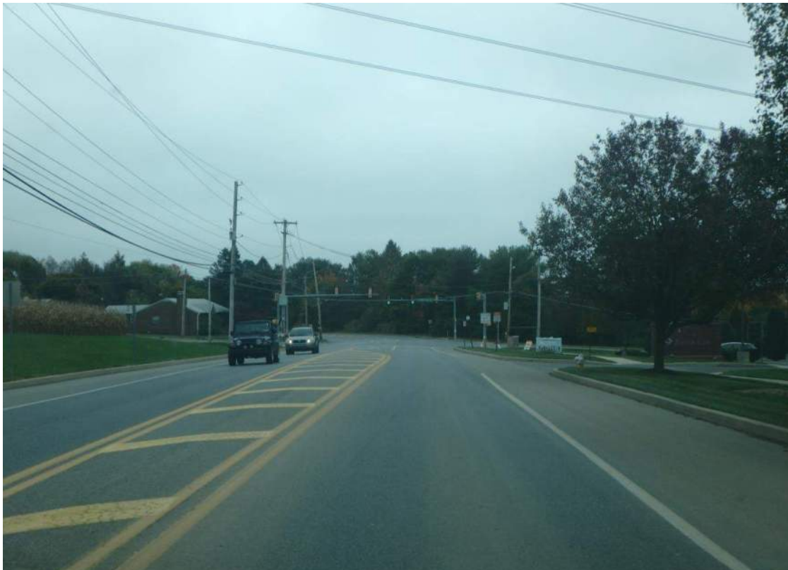
Direction / Road: EB Walbert Ave. Approach / Departure: Approach Distance: 150 Feet
