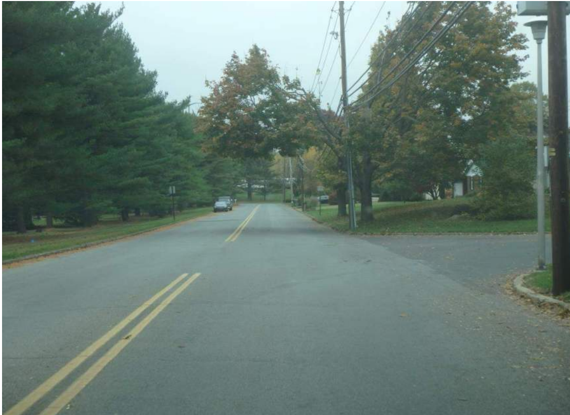
Direction / Road: WB Crackersport Road Approach / Departure: Approach Distance: 50 feet
