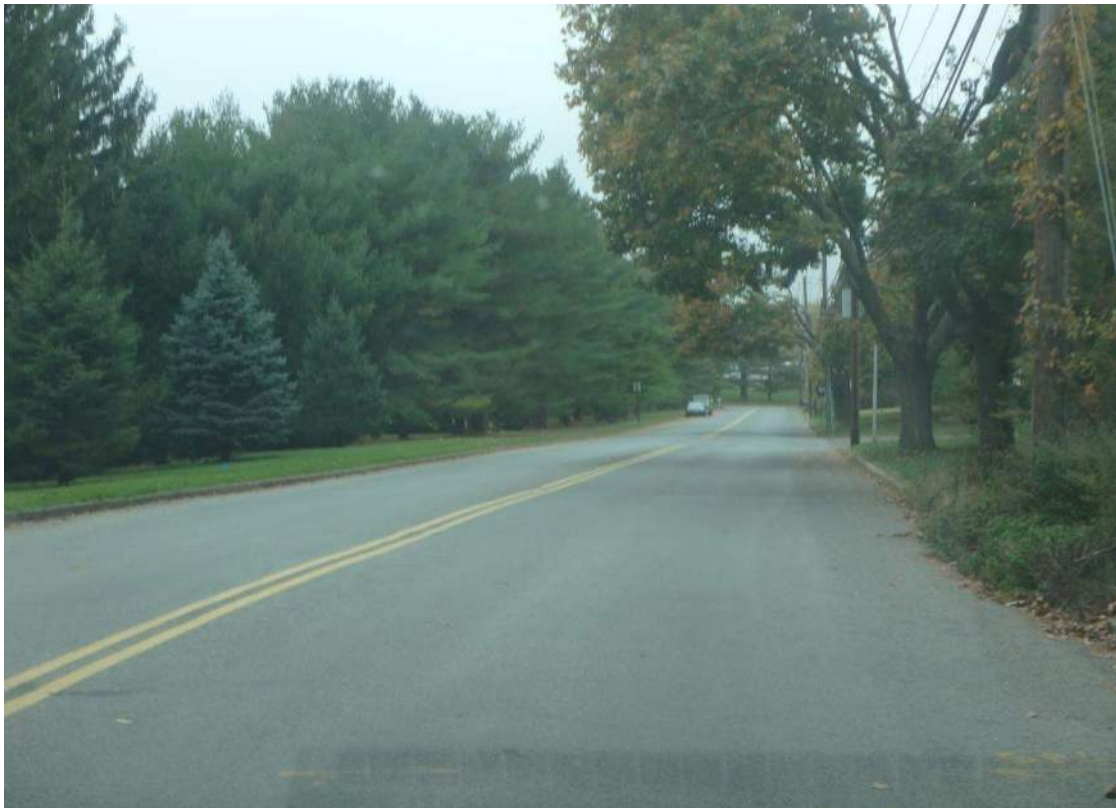
Direction / Road: WB Crackersport Road Approach / Departure: Approach Distance: 150 Feet
