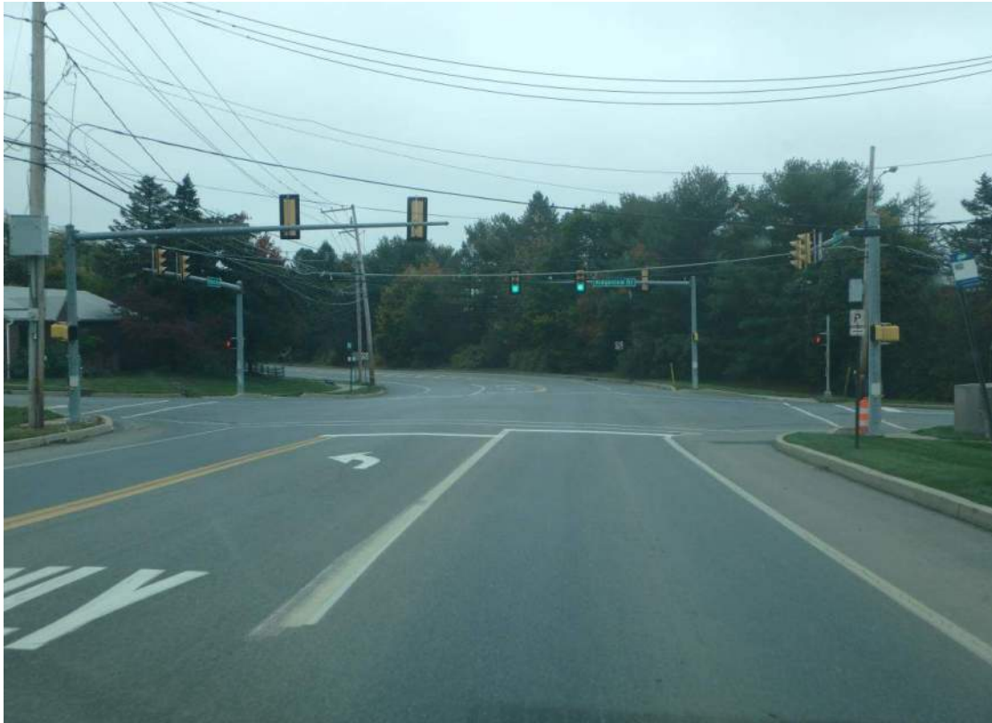
Direction / Road: EB Walbert Ave. Approach / Departure: Approach Distance: 50 feet
