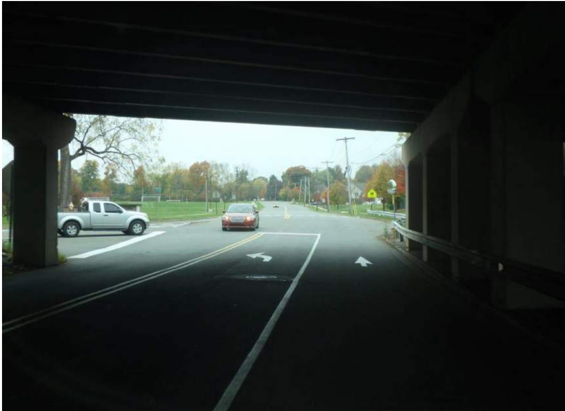
Direction / Road: NB Springhouse Road Approach / Departure: Approach Distance: 50 feet
